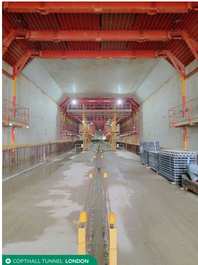
COPTHALL TUNNEL LONDON
